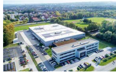
Hesse Mechatronics currently employs around 220 employees in Germany, Hong Kong, Japan and the United States. The headquarters at Lise-Meitner-Straße, completed just three years ago, are now undergoing another several-million-euro expansion.
